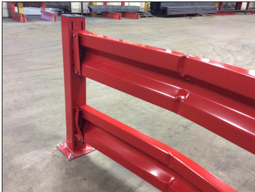
Photo 4: Left side damage to hangers.
