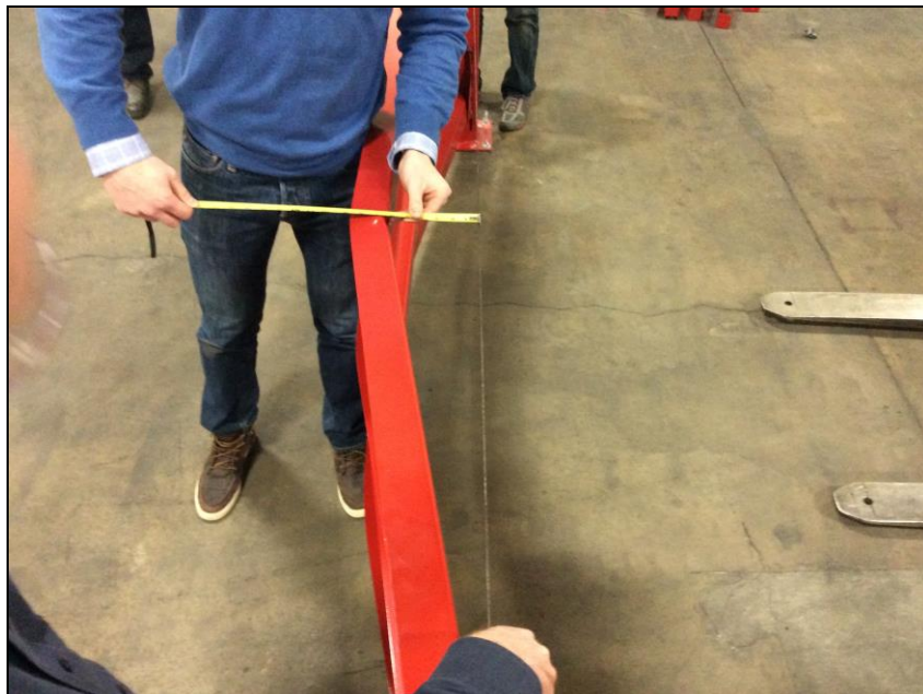
Photo 6: Measurement of deflection at most severe point.
